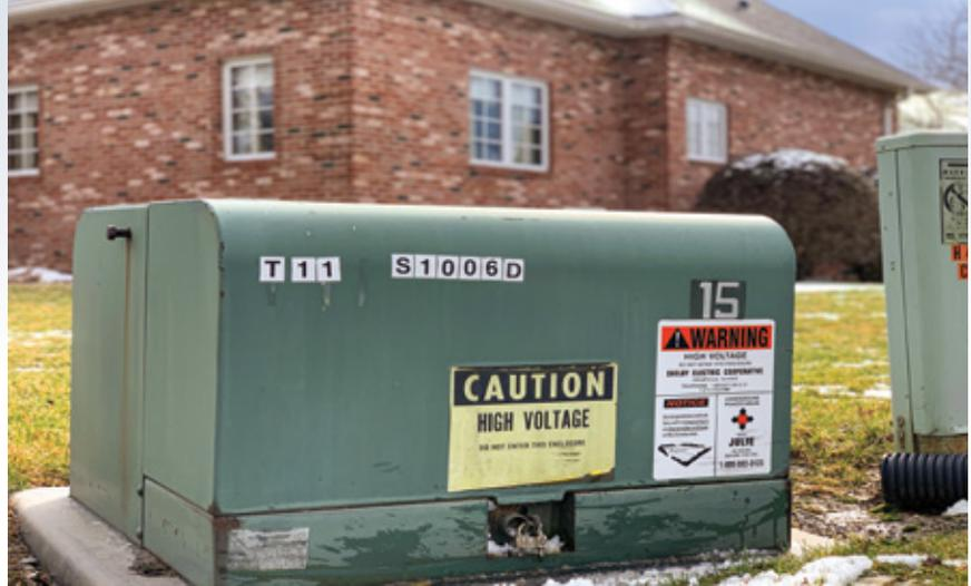
work during an outage and create a serious safety hazard. We need a minimum of 10 feet of clearance in front of the transformer (the side that is padlocked), as well as ample clearance on the other three sides.
